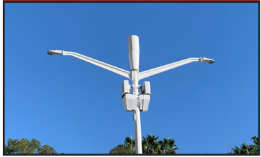
Image Courtesy | Long Beach City website A small cell tower in Long Beach.
