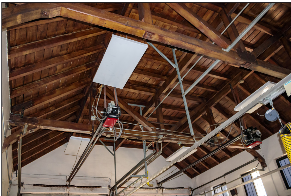
The exposed wooden beams in the truck bay of the former Fire Station 9 building.
