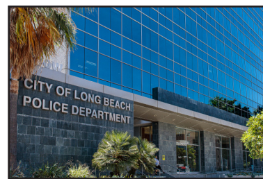
Richard H. Grant | Signal Tribune Exterior picture of the Long Beach Police Department Headquarters in Downtown Long Beach.
