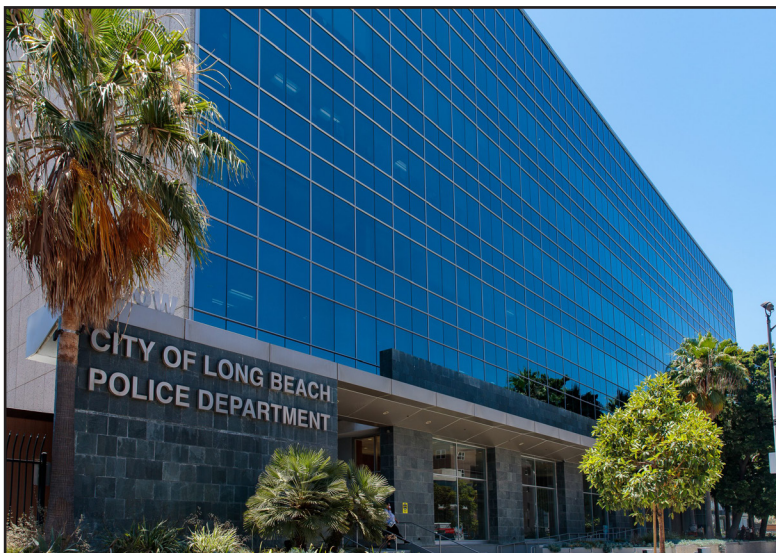
Richard H. Grant | Signal Tribune Exterior view of the Long Beach Police Department Headquarters in Downtown Long Beach
