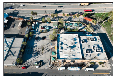
Richard H. Grant | Signal Tribune An aerial view of the Long Beach Multi-Service center on Feb. 6, 2023.
