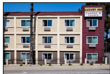
Richard H. Grant | Signal Tribune The exterior of the Luxury Inn motel in North Long Beach on May 9, 2022.
