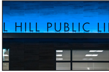
Richard H. Grant | Signal Tribune As part of the recently approved Master Facility Plan, Signal Hill Public Library is slated for a new HVAC system and window repairs.
