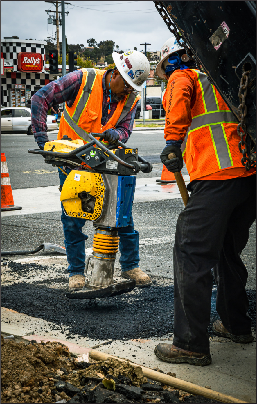
Richard H. Grant | Signal Tribune Construction workers with VCI Construction use a jumping jack tamper to flatten an asphalt patch at Pacific Coast Highway and Cherry Boulevard in Long Beach on May 9, 2023.
