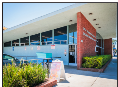
Richard H. Grant | Signal Tribune The Brewitt Library is slated to receive $700,000 in Measure A funds for roof replacement and ancillary repairs.
